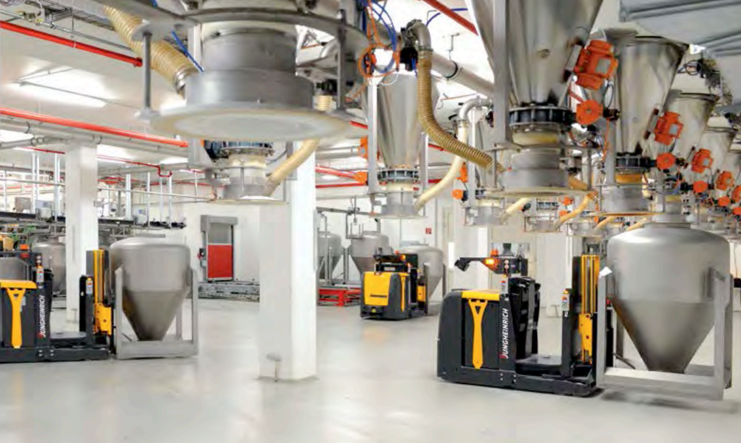
Innovative truck solution: Auto pallet movers enable efficiency increases, as exemplified by the transportation of containers in the silo area of a spice producer.
